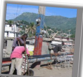
Fig 3b Using electricity from utility pole to arc weld on the side of the street
