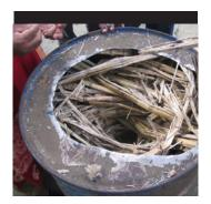
1. Placing bagasse in the oil drum
