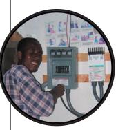
The installation of charge controller and circuit breaker box in a PV system
