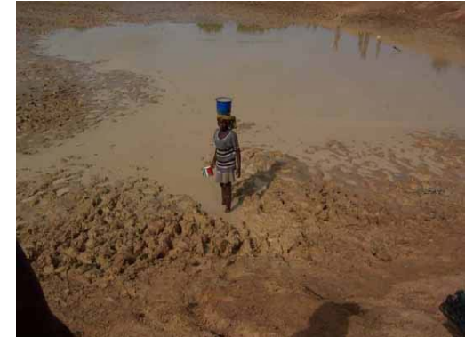
St. Mary's Dam
