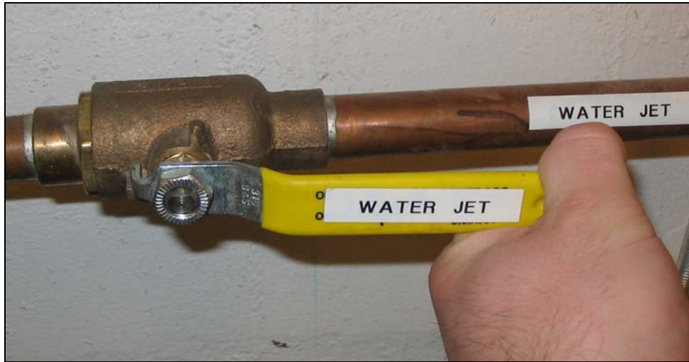
Figure 33 Turning water on/off to water jet cutter
